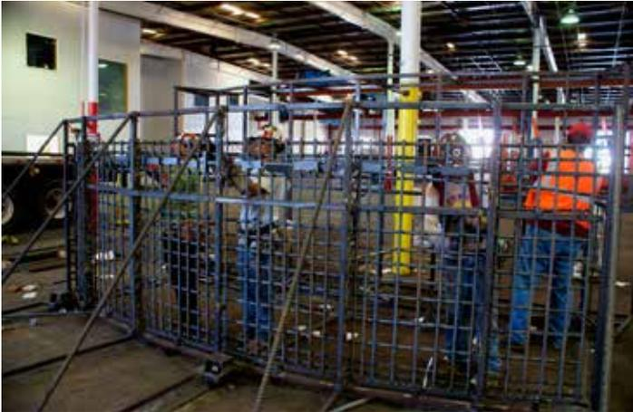
◀ **Assembling segment cages.** Steel Works crews assemble approximately 32 cages daily in a 5mm rotating jig. The bars are cut, bent, and tied into place. After leaving the Steel Works shop, they are placed into molds that form the segments of the tunnel liner.
